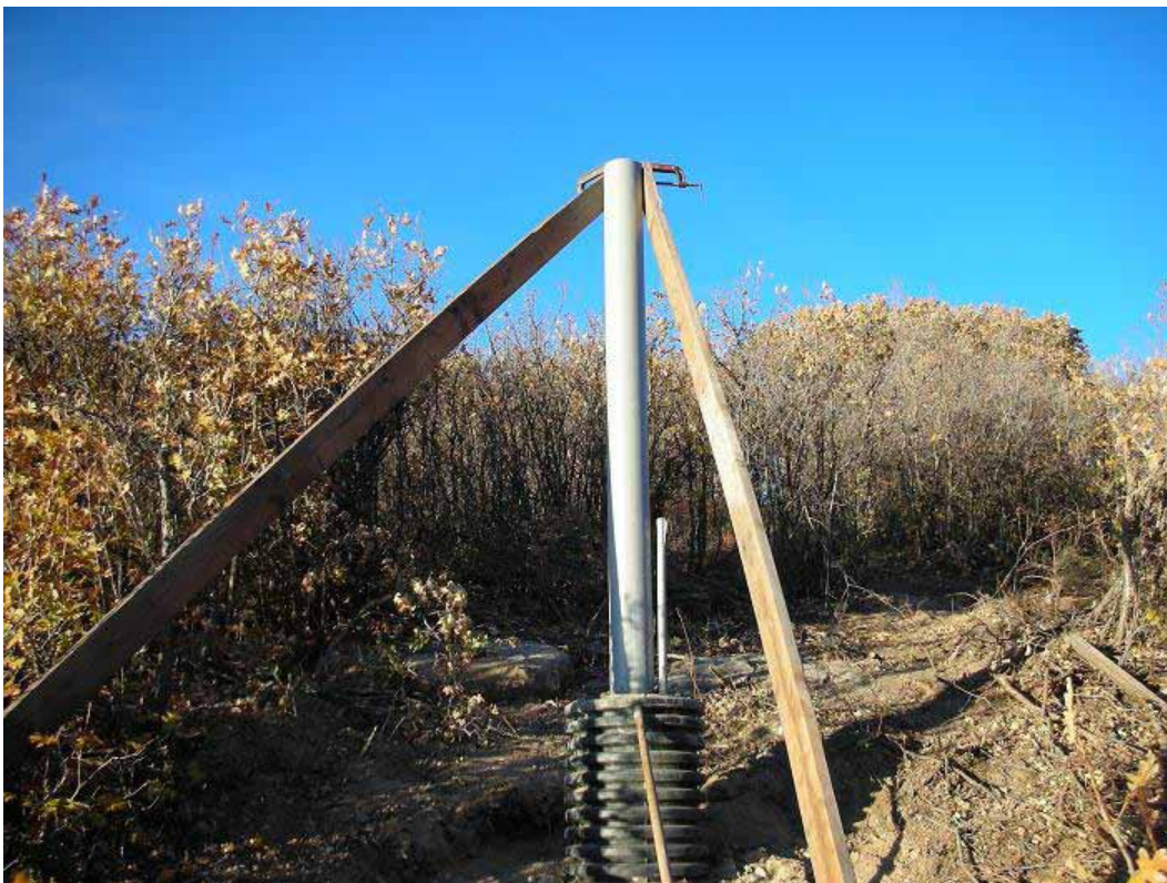
Suggested method of bracing pole plumb before concrete pour.
